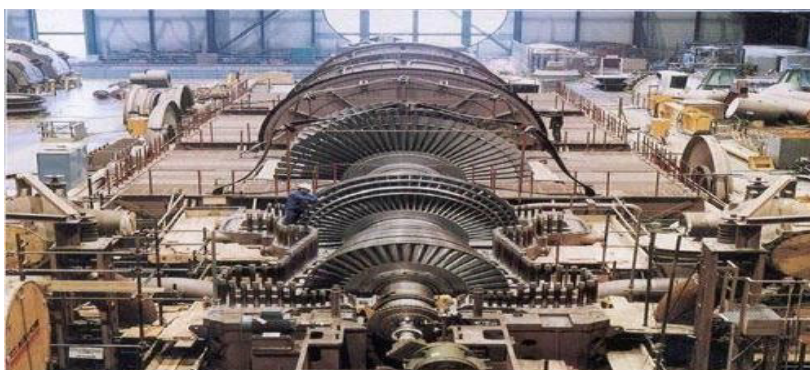
Figure: Steam Turbines
